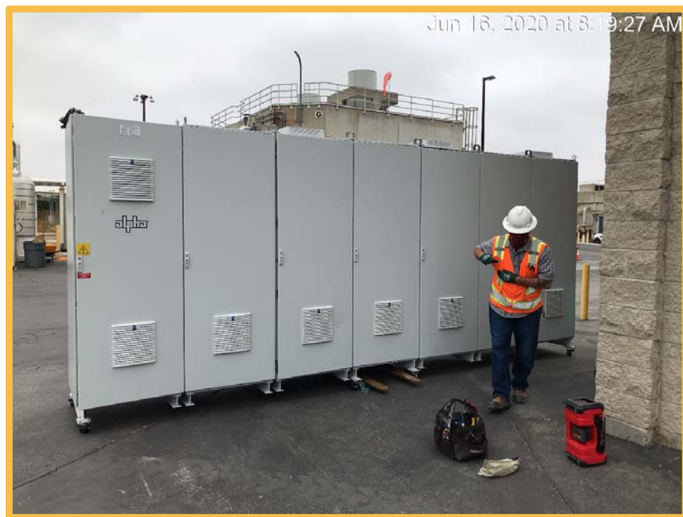
125vDC Battery Cabinets
