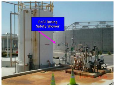
Figure 3-33: Ferric Chloride Dosing Safety Shower
