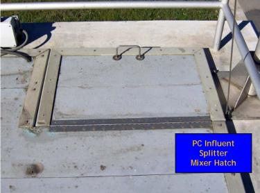
Figure 3-28: Primary Influent Splitter Box Hatch
