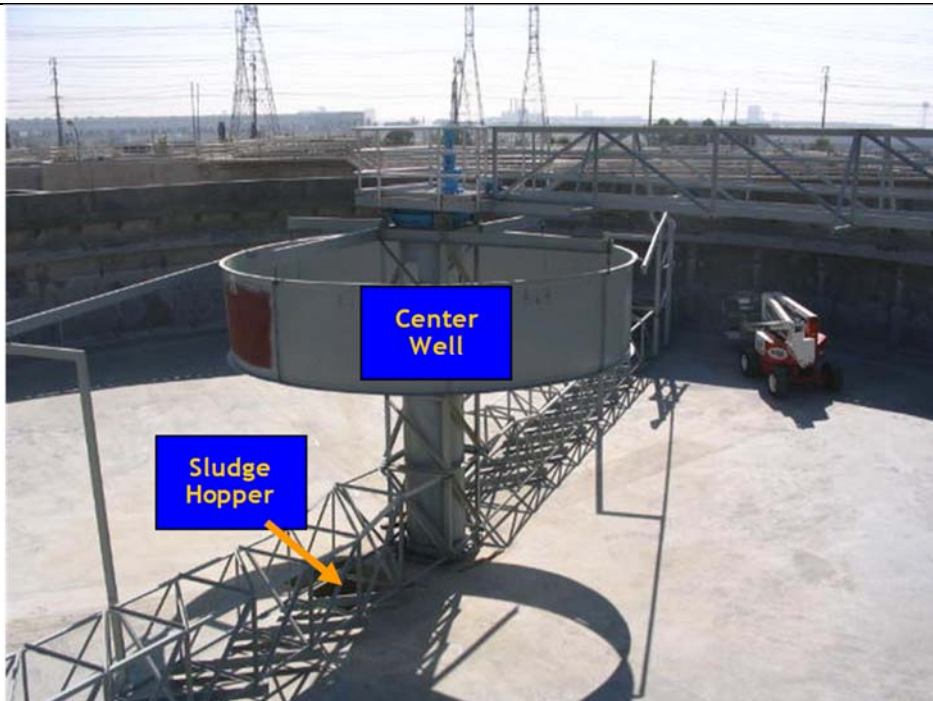
Figure 3-6: Primary Clarifier Stilling Well and Sludge Hopper
