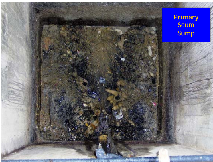
Figure 3-29: Primary Scum Wet-Well
