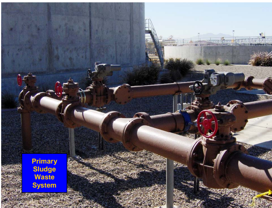
Figure 3-7: Primary Sludge Wasting System
