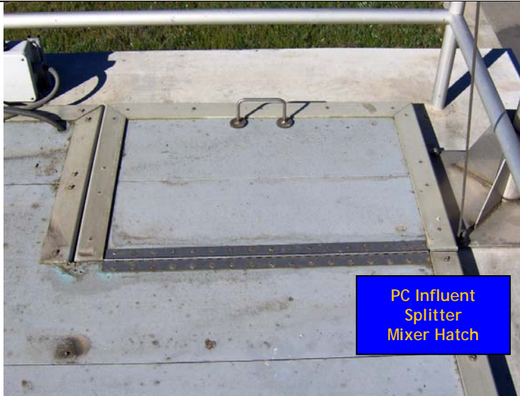
Figure 3-28: Primary Influent Splitter Box Hatch
