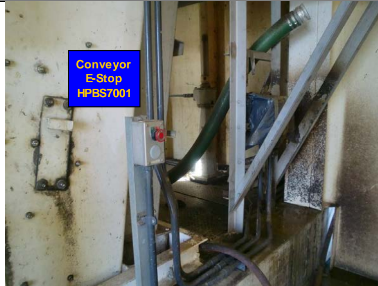
Figure 8: Influent Screen Conveyor E-Stop
