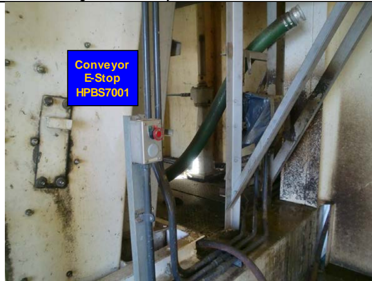
Figure 11: Influent Screen Conveyor E-Stop
