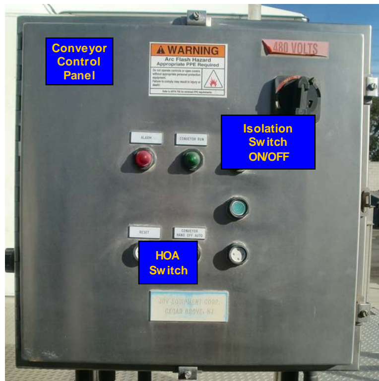
Figure 9: Influent Screen Conveyor Control Panel
