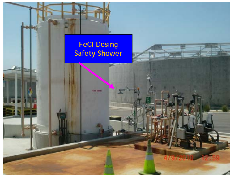
Figure 3-33: Ferric Chloride Dosing Safety Shower
