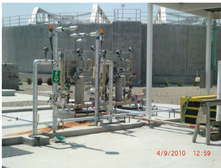
Figure 3-36: Polymer Dosing Safety Shower
