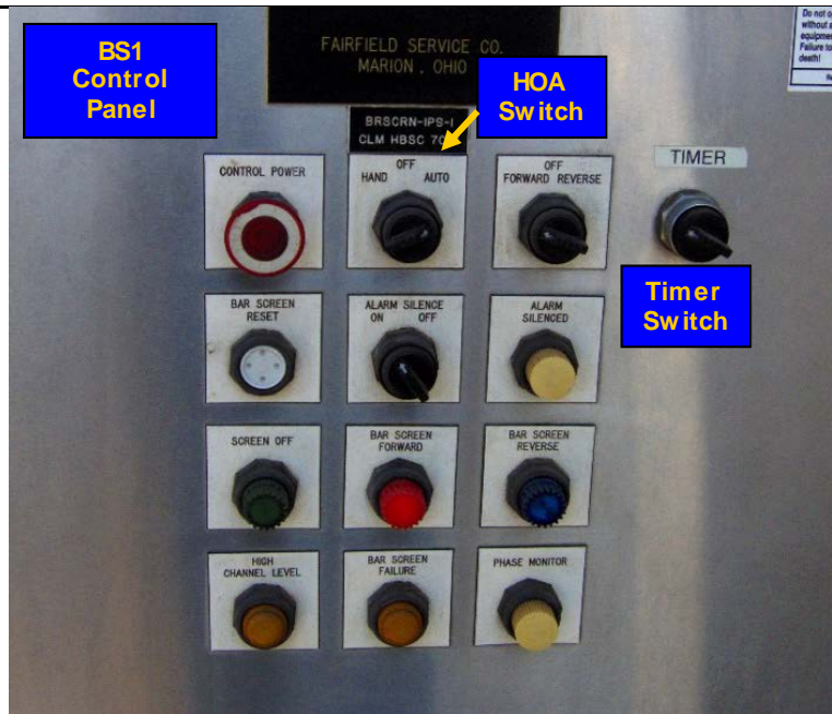
Figure 12: Influent Screen#1 Local Control Panel The screen will now start via an electro-mechanical timing signal located in the Local Control Panel. Once started, the rake carriage will start its run cycle.
