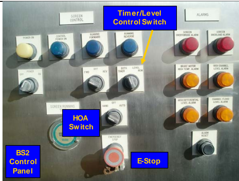
Figure 13: Influent Screen#2 Local Control Panel The screen will now start via a timing signal from a PLC located in the Local Control Panel. Once started, the rake carriage will start its run cycle. If the initiating contact
