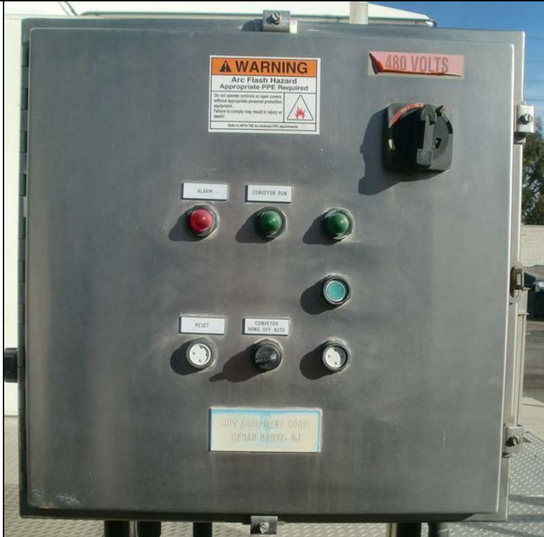
Figure 17: Influent Screen #2 Local Control Panel
