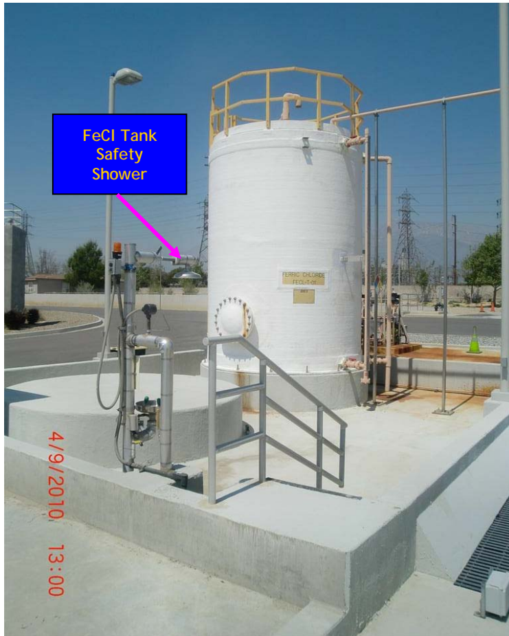
Figure 3-35: Ferric Chloride Tank Safety Shower
