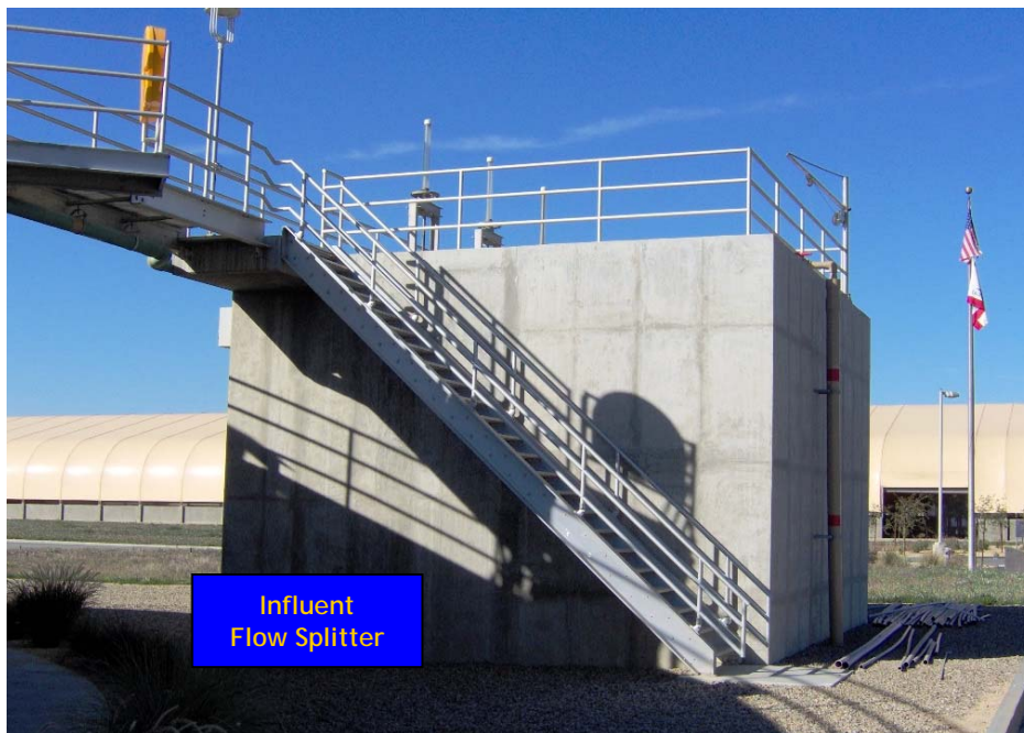
Figure 3-1: Primary Influent Flow Splitter Structure
