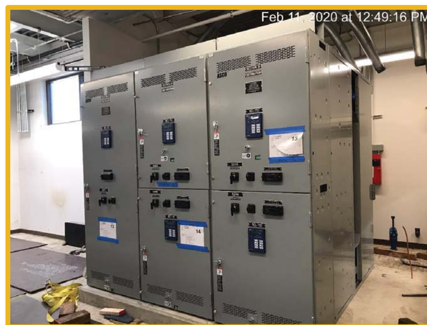
RP-1 12kV Switchgear Extension
