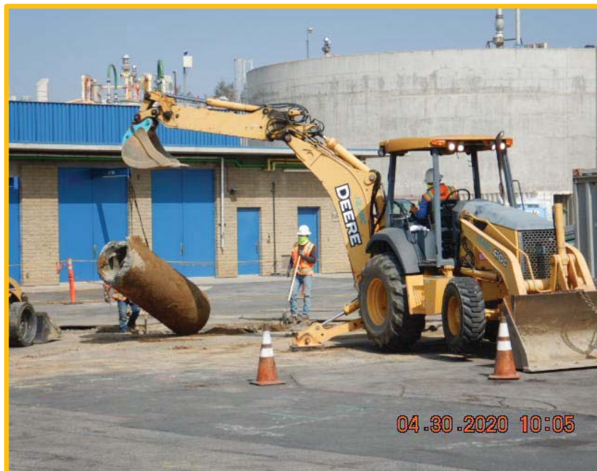
Clearing 27-in Abandoned Pipeline
