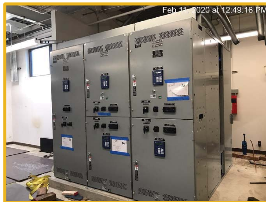
RP-1 12kV Switchgear Extension
