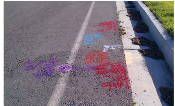
Marked Recycled and Potable Water
