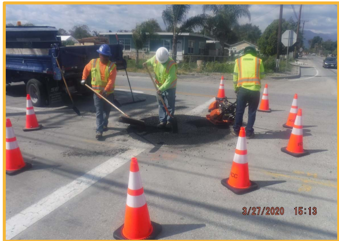
Placing Asphalt
