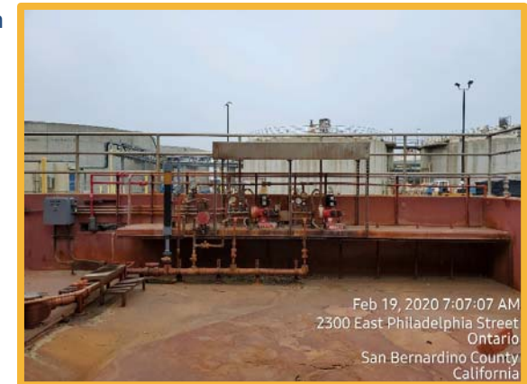
RP-1 Ferric Chloride Station
