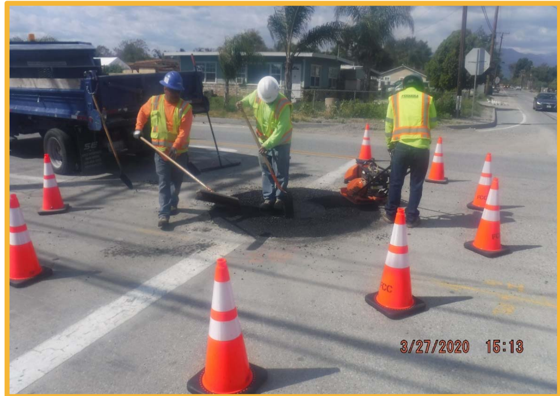
Placing Asphalt
