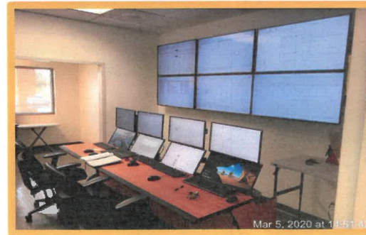
Upgraded Control Rooms
