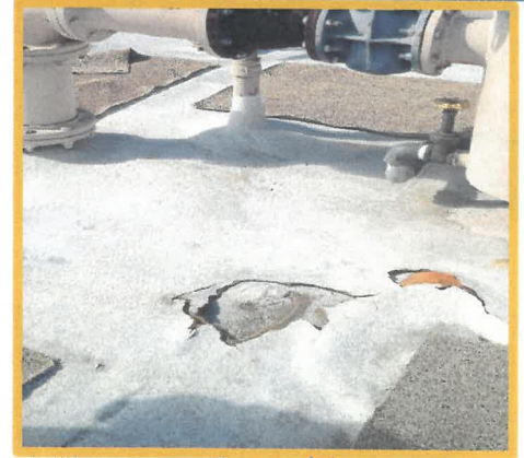
Cracking of Foam Roofing Insulation
