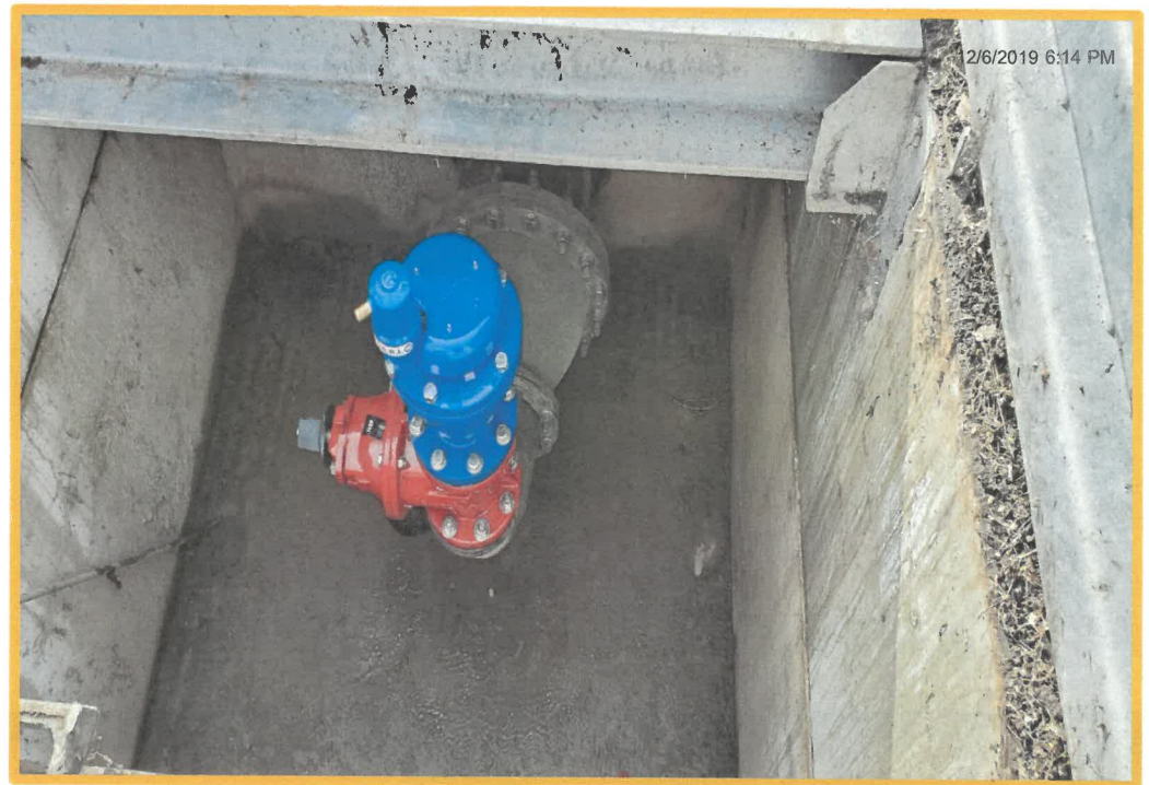
New Air Release Valve in Vault
