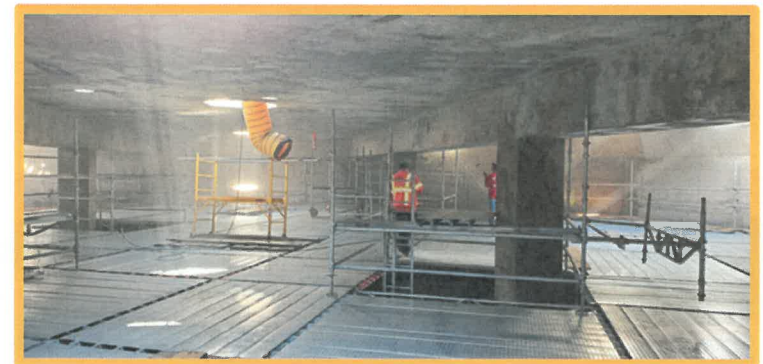
Digester Scaffolding and Coating
