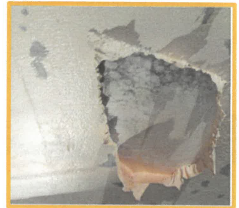
Failed Internal Roof Coating
