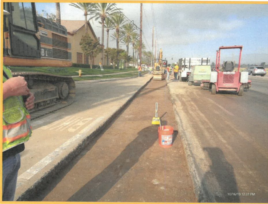
Base Paving After Pipe Installation
