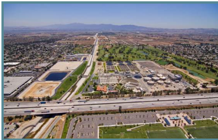
Regional Water Recycling Plant No. 1 (RP-1)
