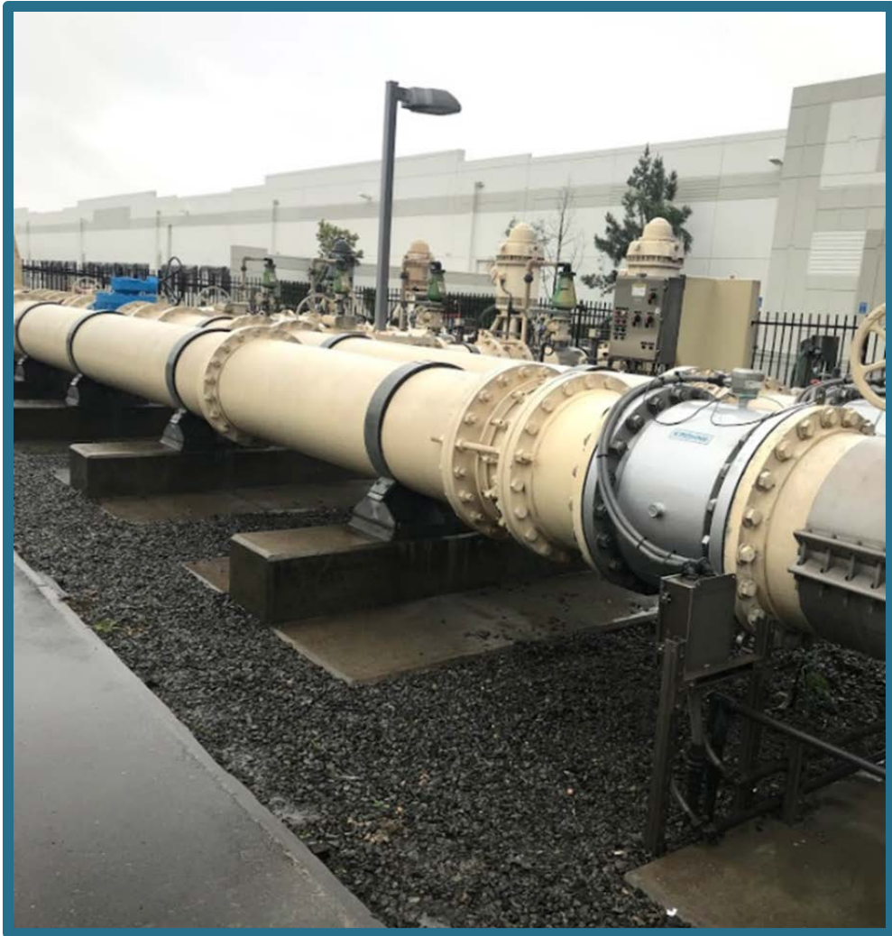
Lift Station Force Mains and Meters
