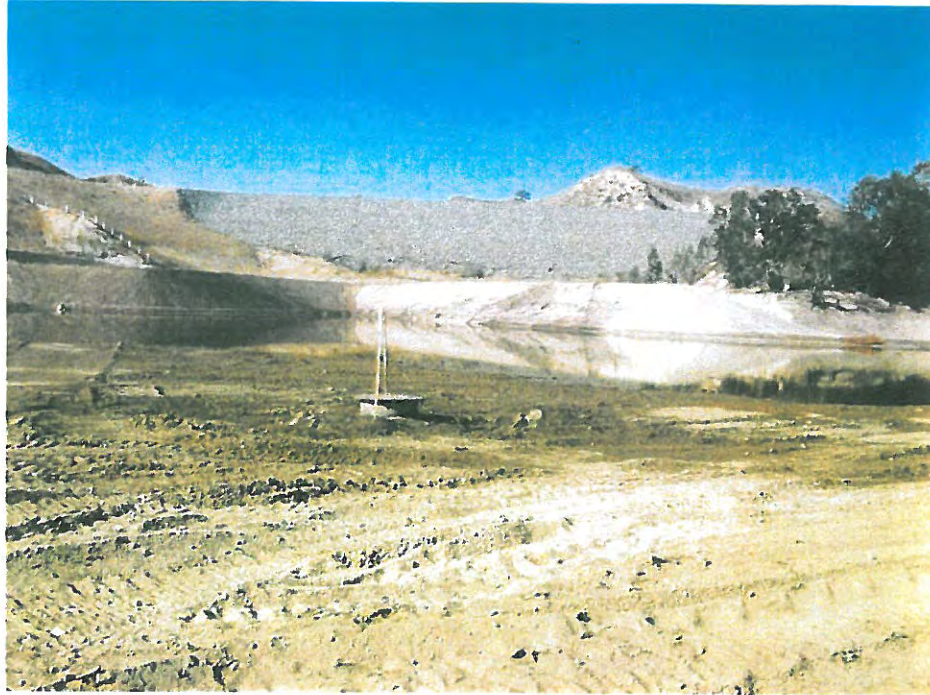
Photo 1. Looking at manhole 4A-0000 near dam inlet within inundation area.
