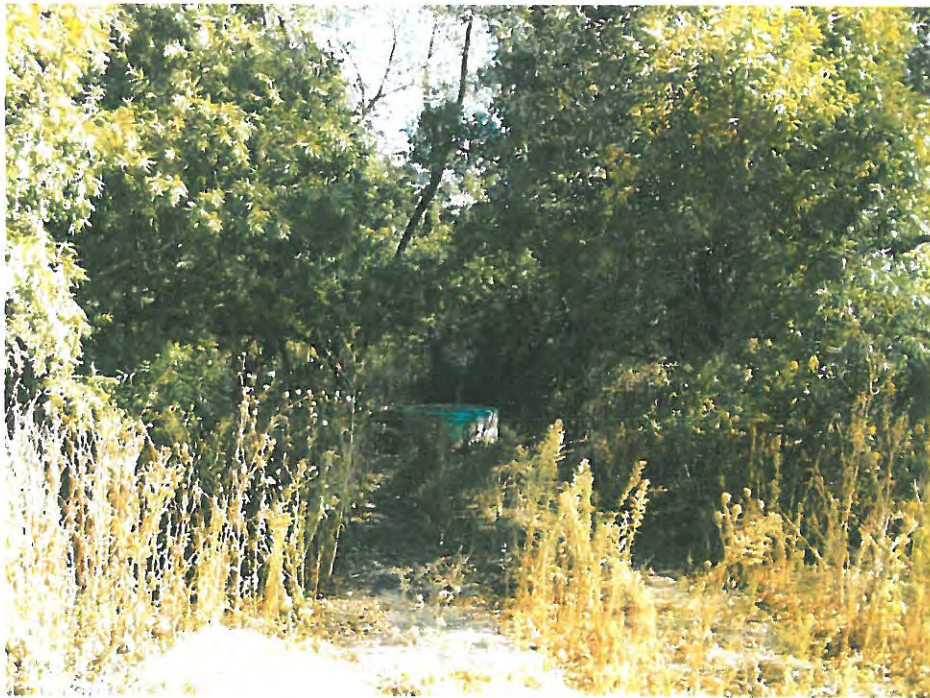
Photo 22. Looking at manhole 4A-0090.
