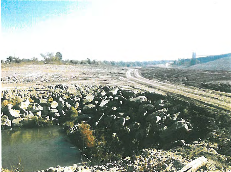
Photo 3. Near manhole 4A-0000 and 4B-0010.
