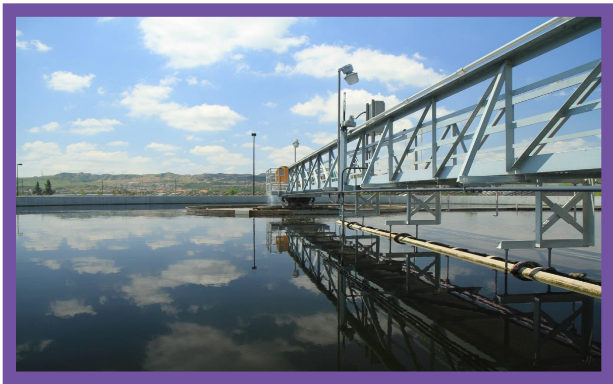
REGIONAL WATER RECYCLING PLANT NO. 5 SECONDARY CLARIFIER
