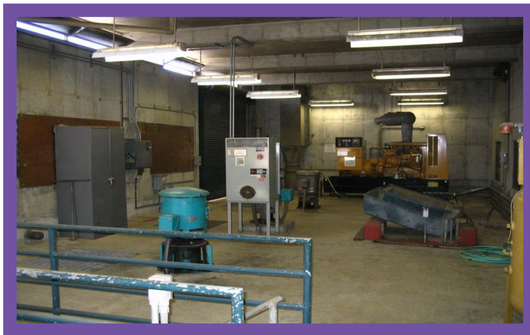
PHILADELPHIA LIFT STATION
