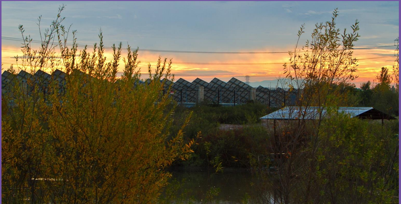
REGIONAL WATER RECYCLING PLANT NO. 5 – SOLAR PANELS
