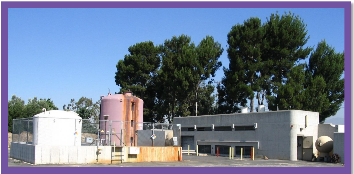
PHILADELPHIA LIFT STATION
