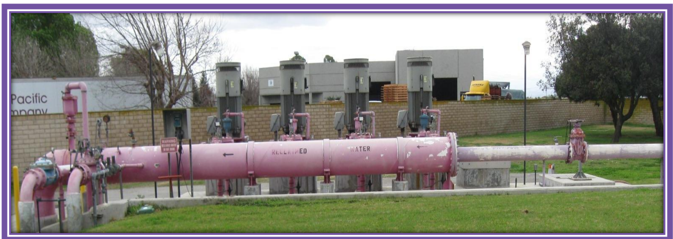
CCWRF Recycled Water Pump Station – Chino, CA
