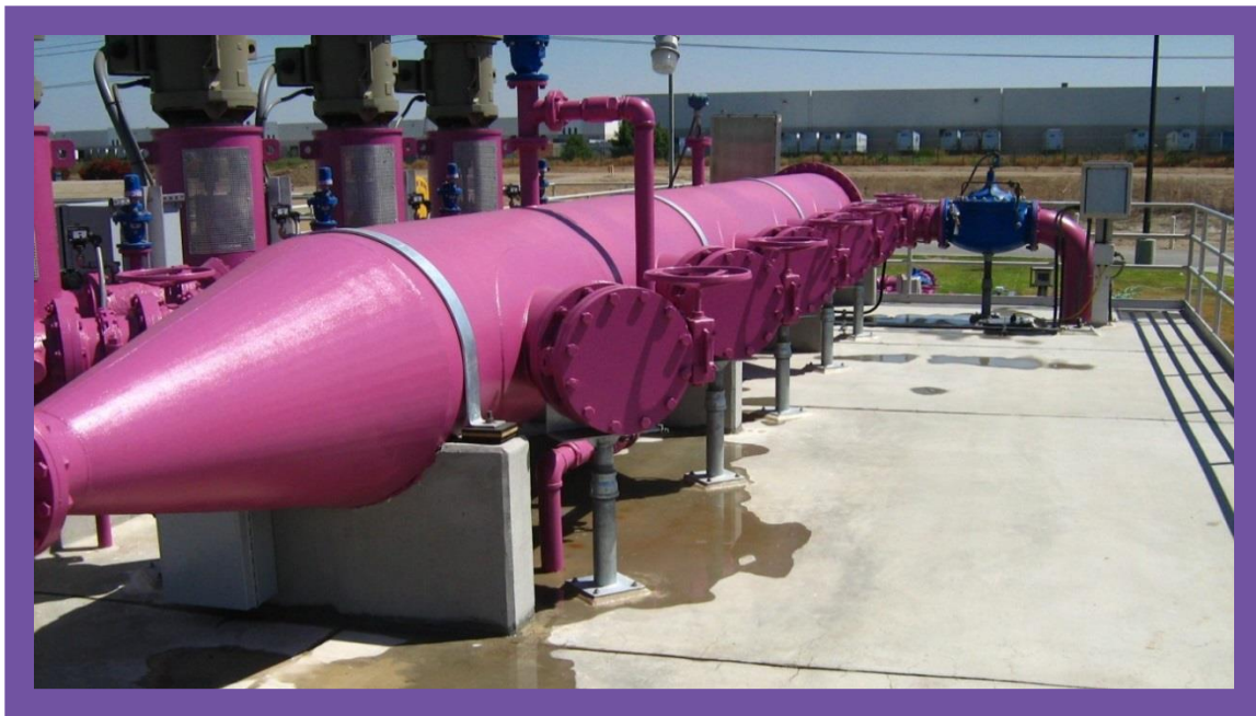
REGIONAL WATER RECYCLING PLANT NO. 5 RECYCLED WATER PUMP STATION
