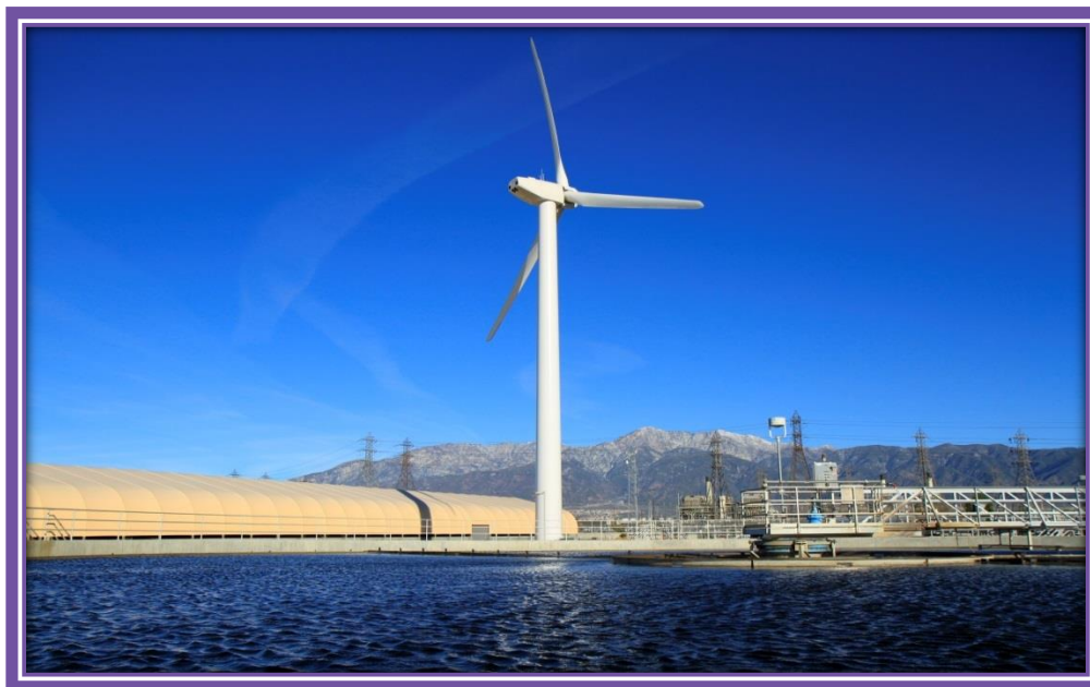
REGIONAL WATER RECYCLING PLANT NO. 4 – WIND TURBINE
