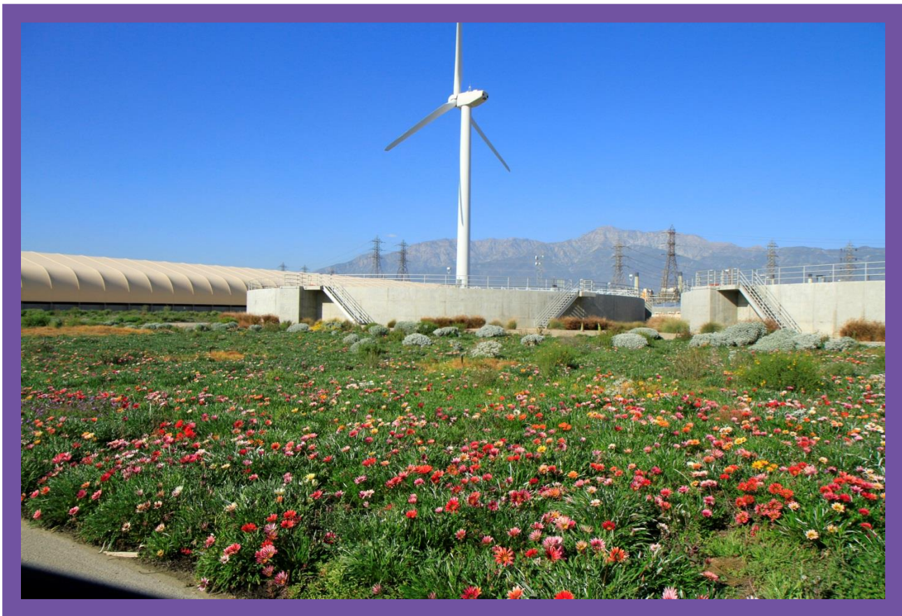
REGIONAL WATER RECYCLING PLANT NO. 4
