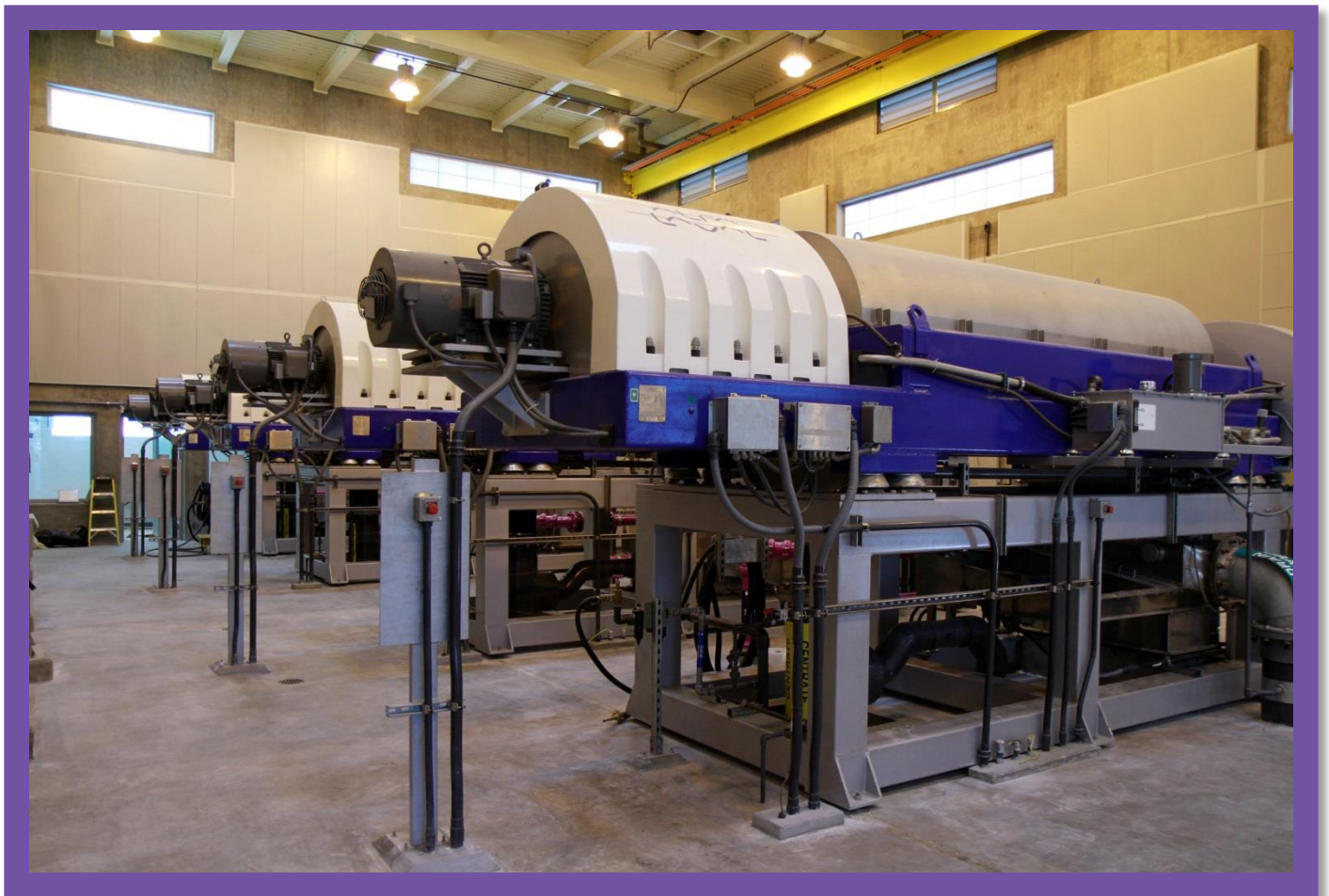
REGIONAL WATER RECYCLING PLANT NO. 1 - DEWATERING
