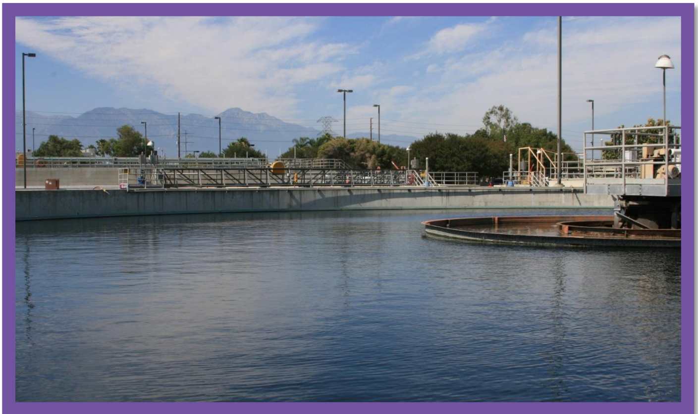
CARBON CANYON WATER RECYCLING FACILITY
