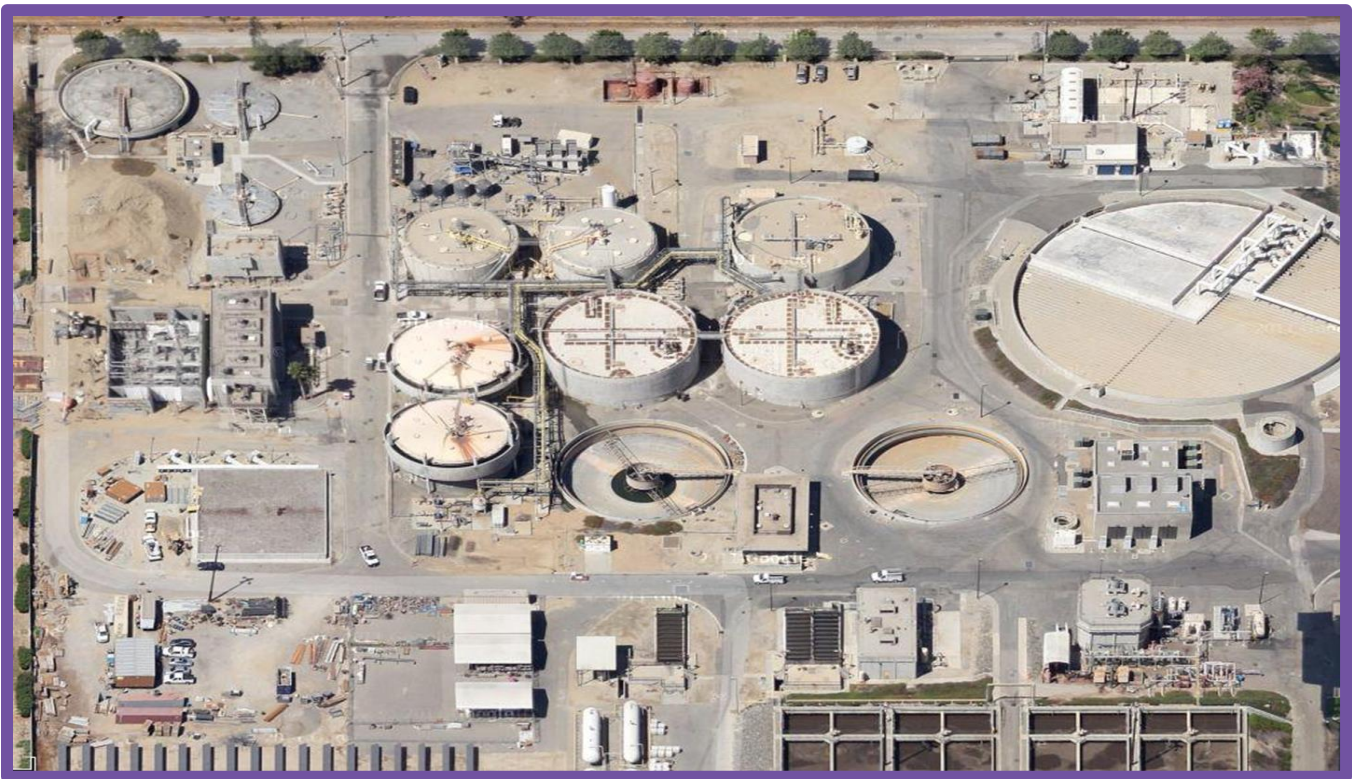
RP-1 AERIAL VIEW
