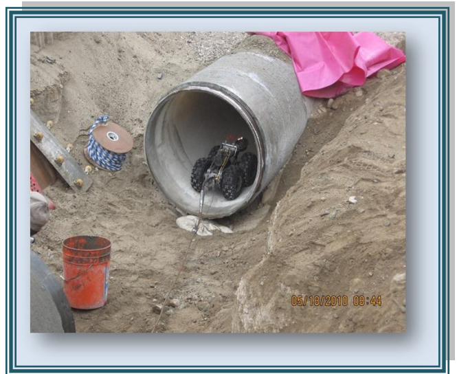
36" Recycled Water Pipeline Performing Camera Survey
