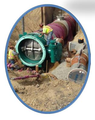
The layout of the proposed lots and streets in the proposed residential development in the City of Ontario (between Riverside Drive and Chino Avenue), the existing 30-inch RP-1 Outfall recycled water pipeline needed to be relocated outside of its easement into public right-of-way. Two 72-inch triple offset butterfly valves were installed.
