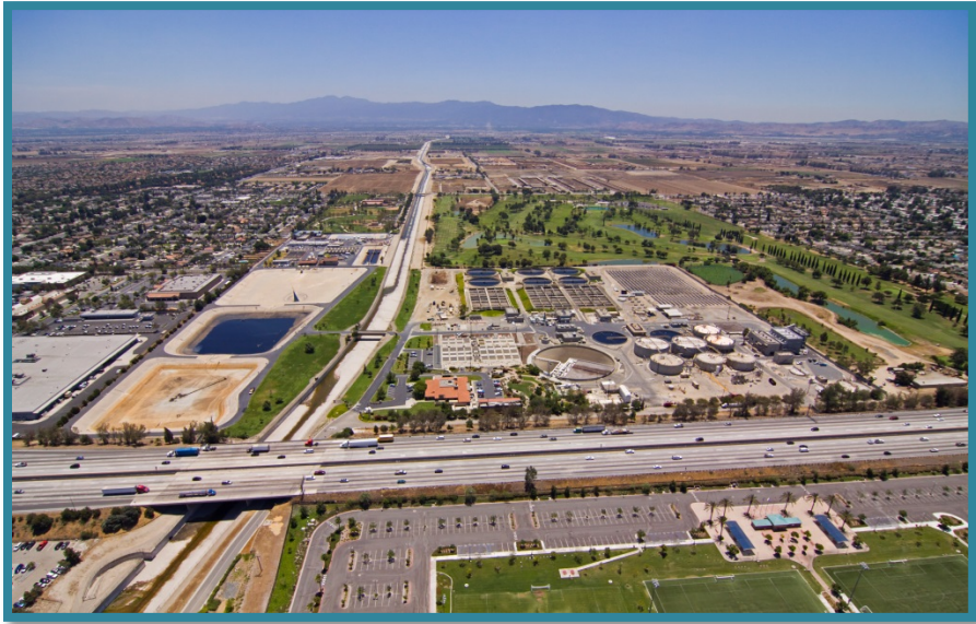
Regional Water Recycling Plant No. 1 (RP-1)
