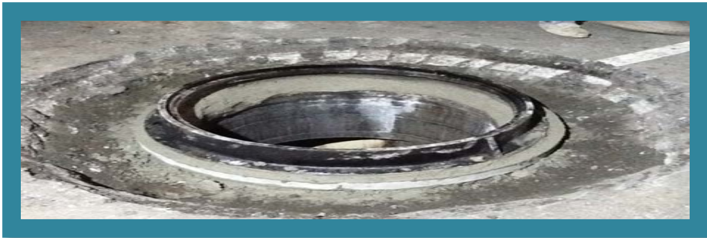
NRW Collection System Repair – Sewer Manhole
