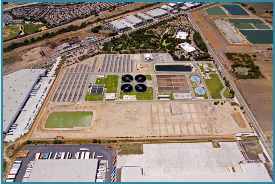
Regional Water Recycling Plant No. 5 (RP-5)
