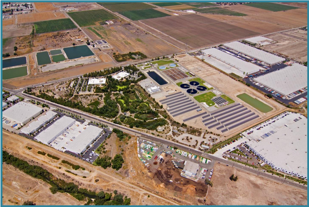
IEUA Headquarters/Regional Water Recycling Plant No. 5
