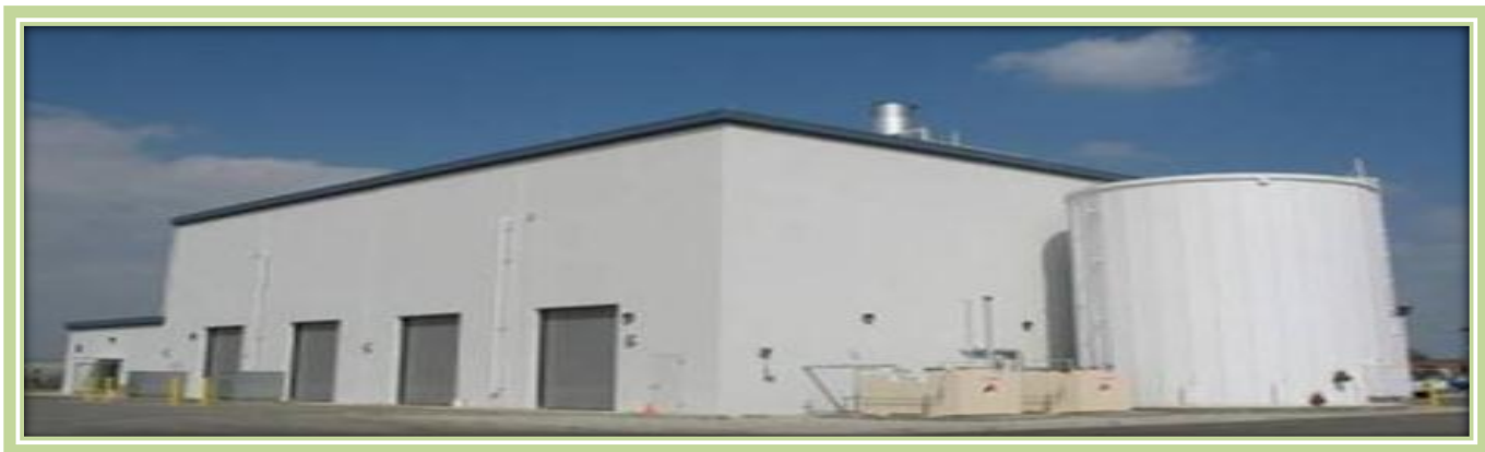
Renewable Energy Efficiency Facility (REEP) – Chino, CA
