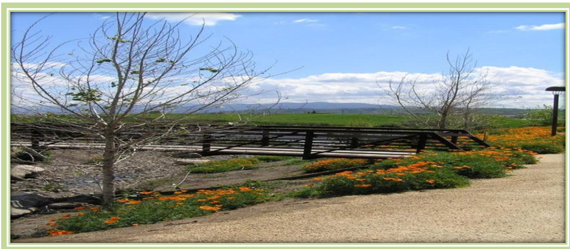
IEUA Headquarters Bridge - Chino, CA
