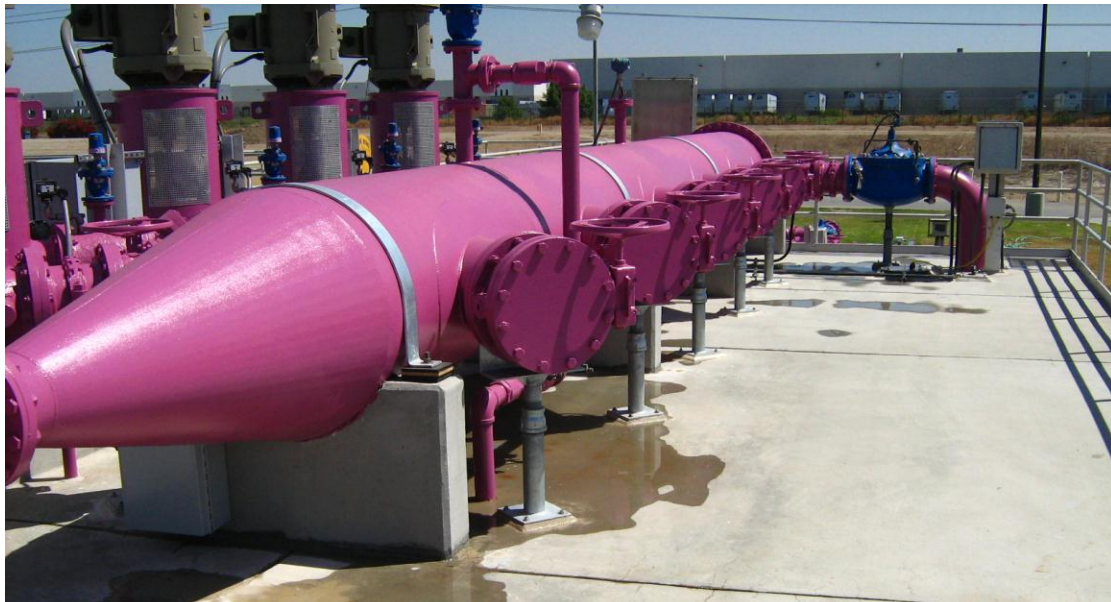
Regional Plant No. 5 Recycled Water Pump Station
