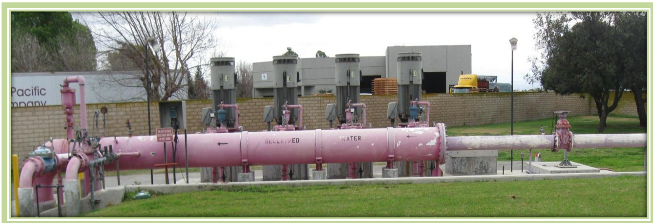
CCWRF Recycled Water Pump Station – Chino, CA
