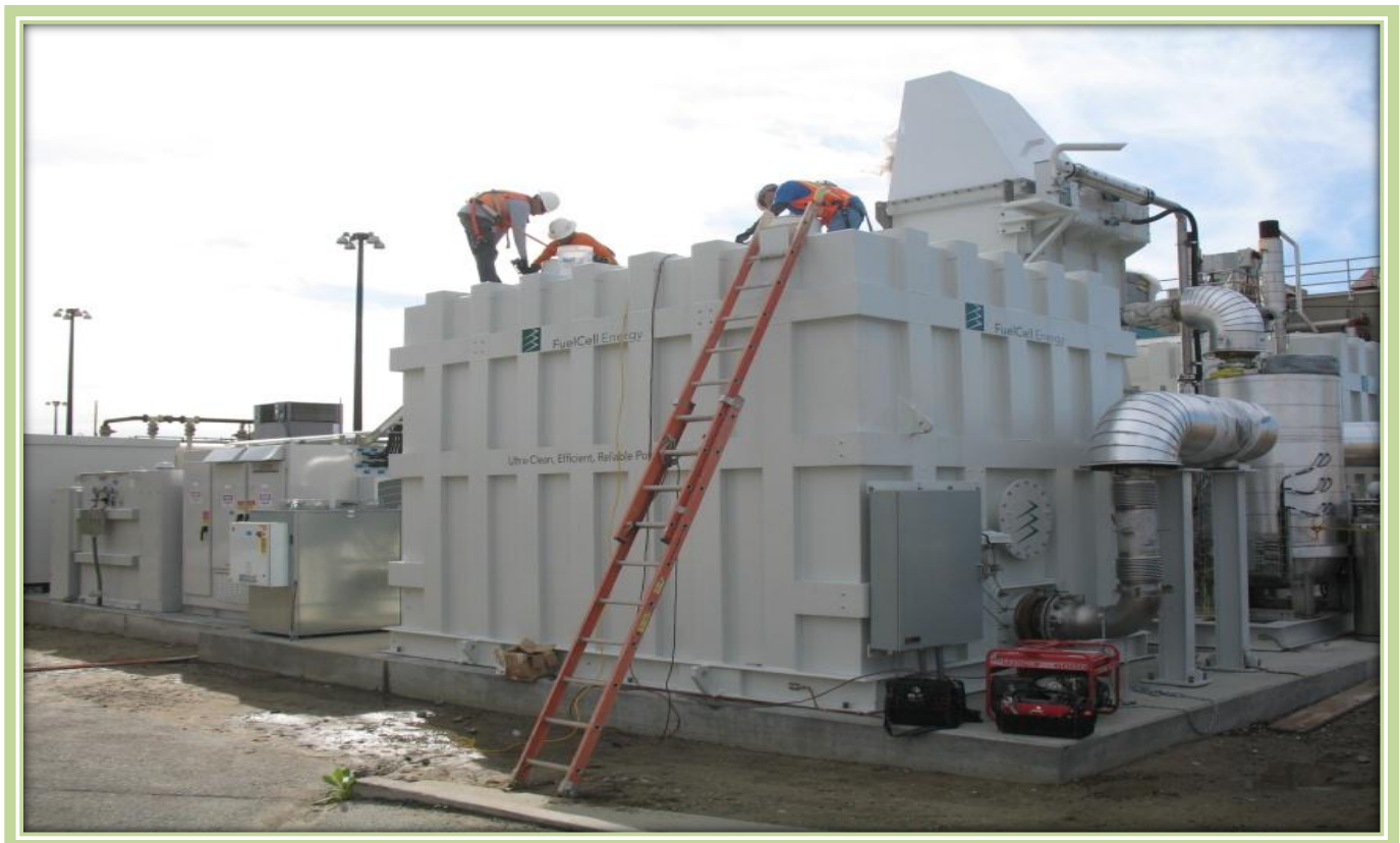
Fuel Cell Project – Regional Plant No. 1 – Ontario, CA
