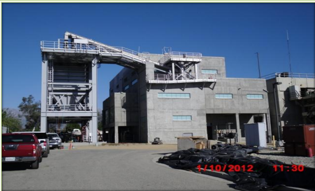
Regional Plant No. 1 – Ontario, CA
