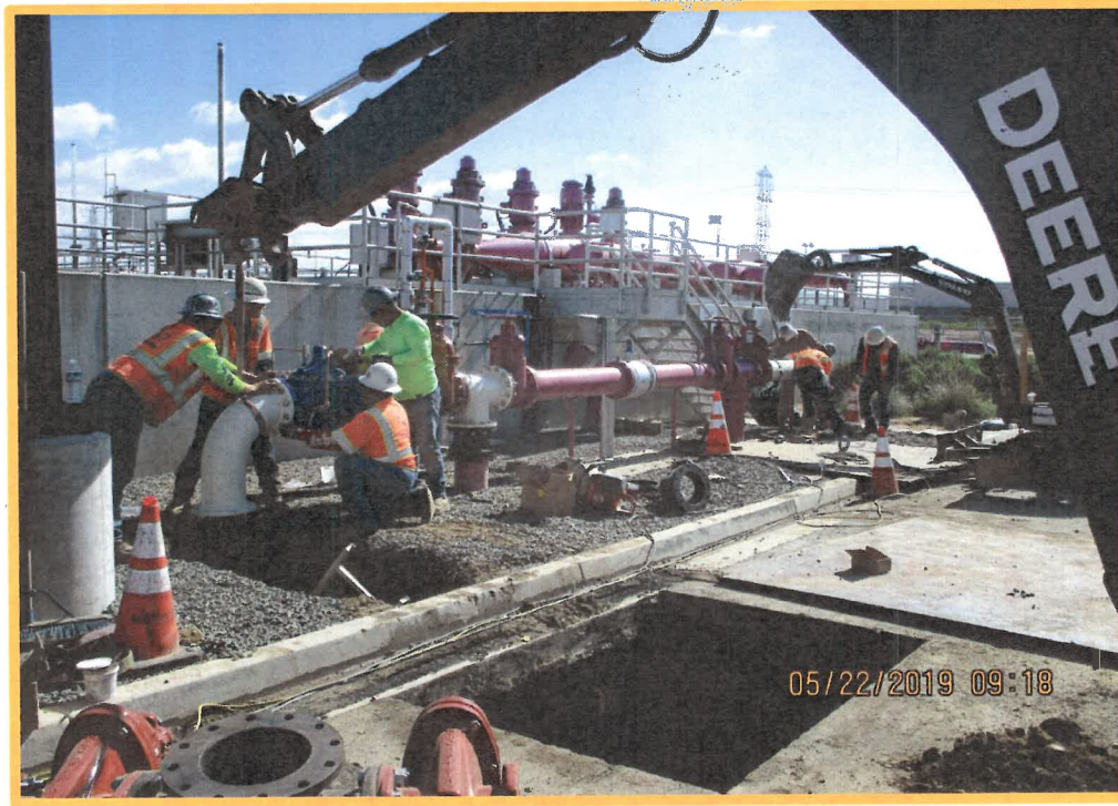
Piping Upgrade in Progress
