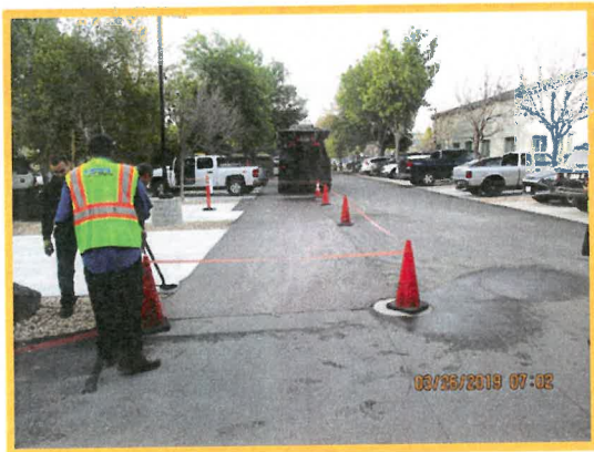
HQ Paving Safety Improvements
