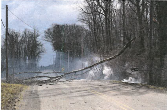
Trees Falling Onto Power Lines
