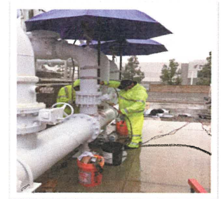
CDA Winter Maintenance Shutdown
