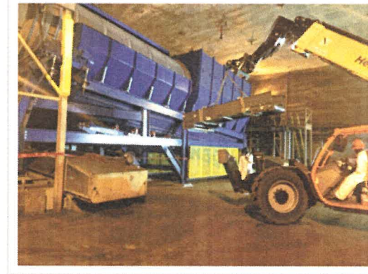
IERCF Compost Screening Replacement
