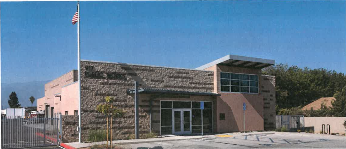
built- San Gabriel Municipal Yard
