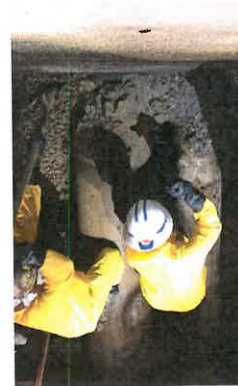
Engineering: Pipeline Repair
