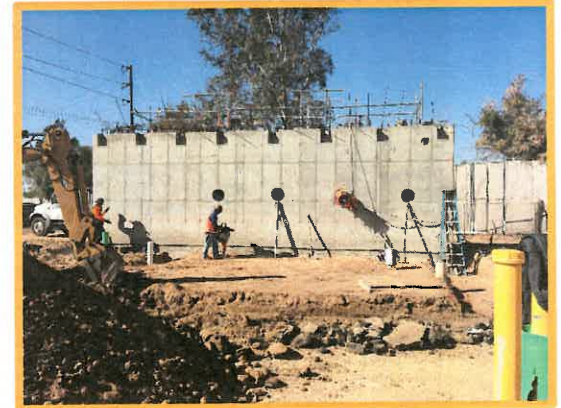
Wet Well Construction
