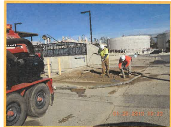
Potholing for Scum Piping
