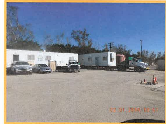
Contractor Mobilization at RP-1 Headworks
