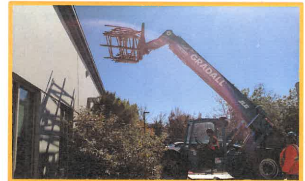
Moving Materials to Roof
