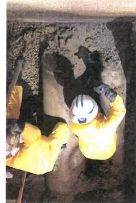
Engineering: Pipeline Repair
