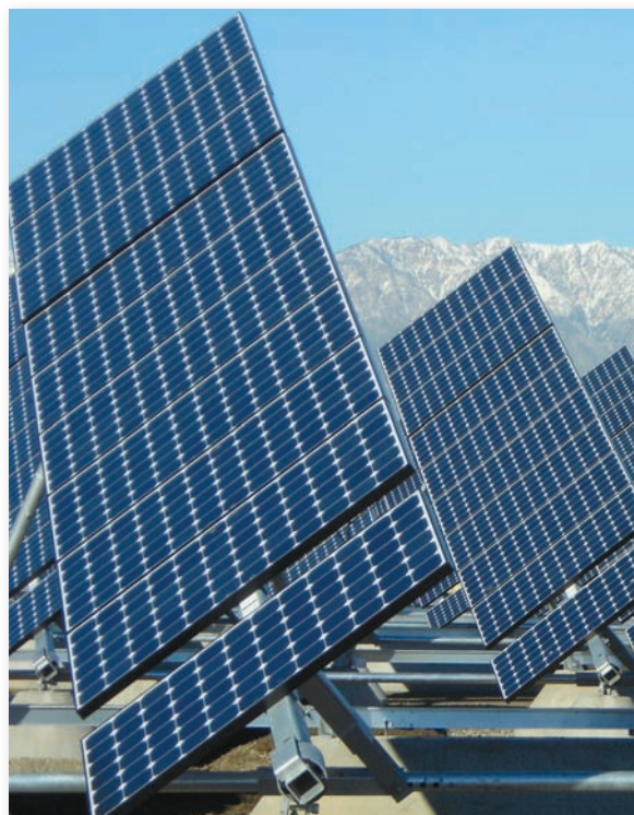
Solar panels provide nearly 100% of peak power demands at IEUA's Regional Water Recycling Plant No. 5.
