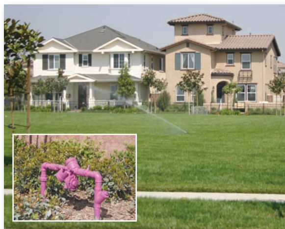
Purple pipes indicate recycled water which is used to water golf courses, medians and parks.
