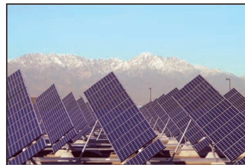
The newly constructed solar power system will save IEUA more than $300,000 per year in electrical costs.
