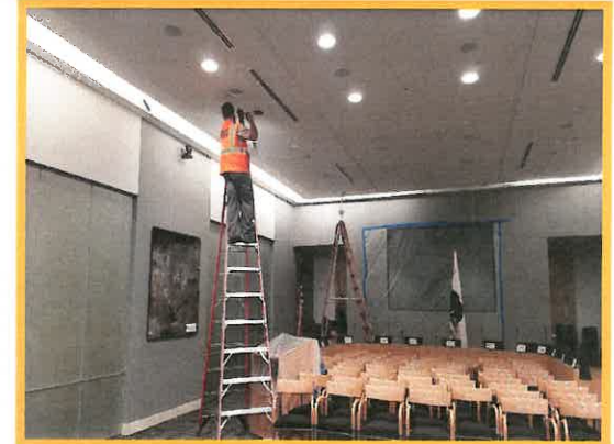
Installing New Lights in Boardroom at HQ-A
