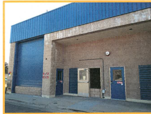
Current Access to Chemical Building
