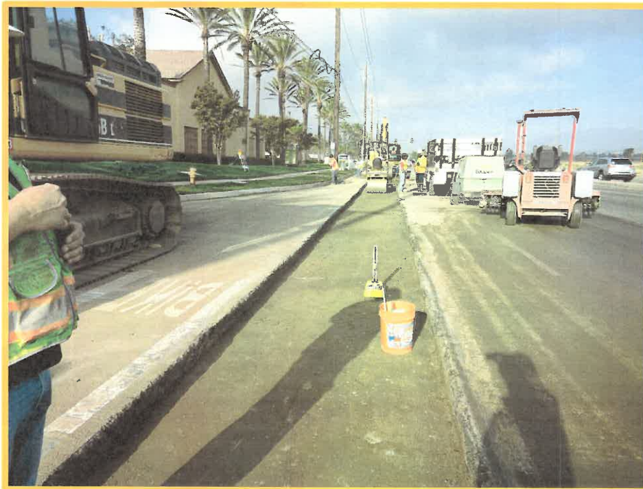
Base Paving After Pipe Installation
