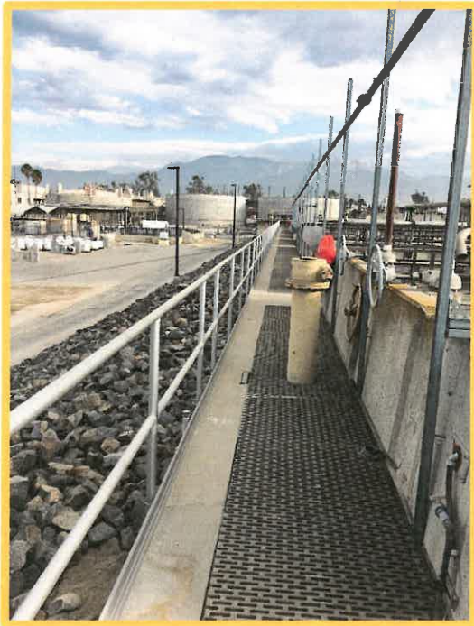
Aeration Basin Railing Installed
