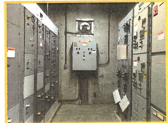
Existing Motor Control Center
