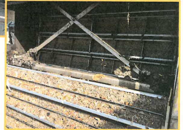
Rag Accumulation Inside Fine Screens
