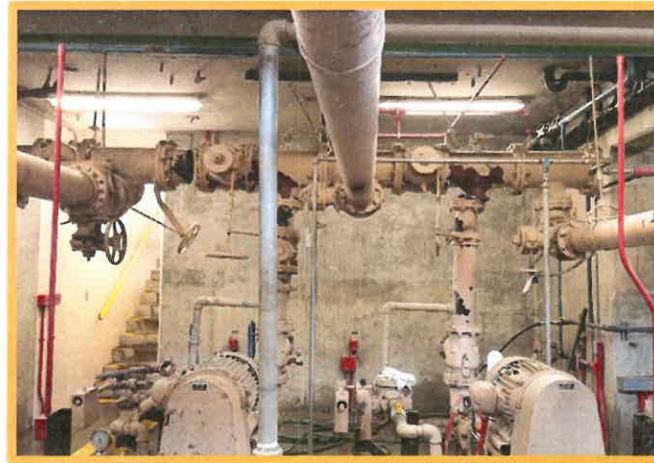
Ruptured Primary Sludge Piping
