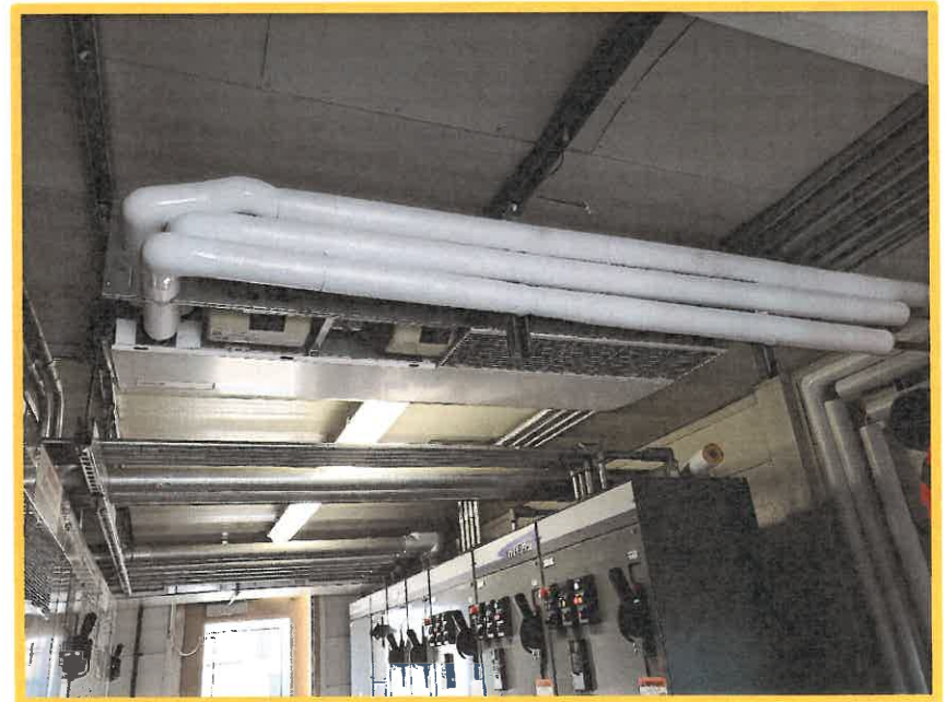
New Ductless Fan Coil with Insulated Electrical Conduits
