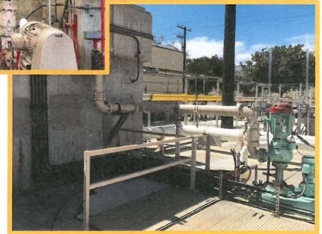
Grit Pump Discharge Pipeline
