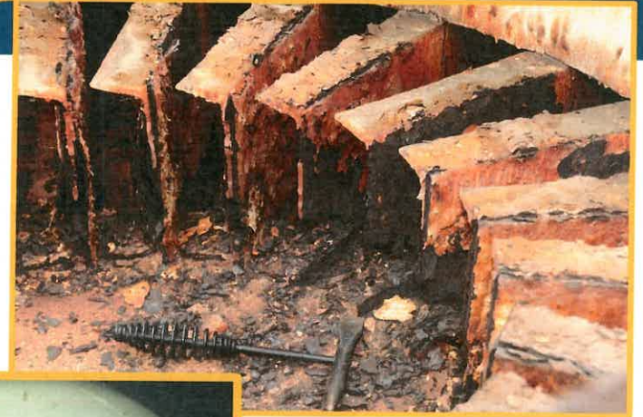
Corrosion Damage on Rafters
