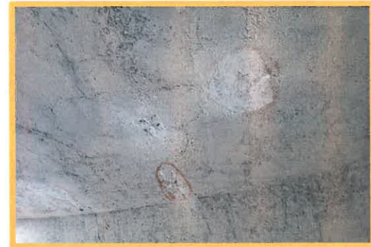
Sample Roof Sand Blasted Area
