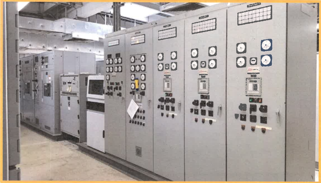
RP-1 Emergency Generators
