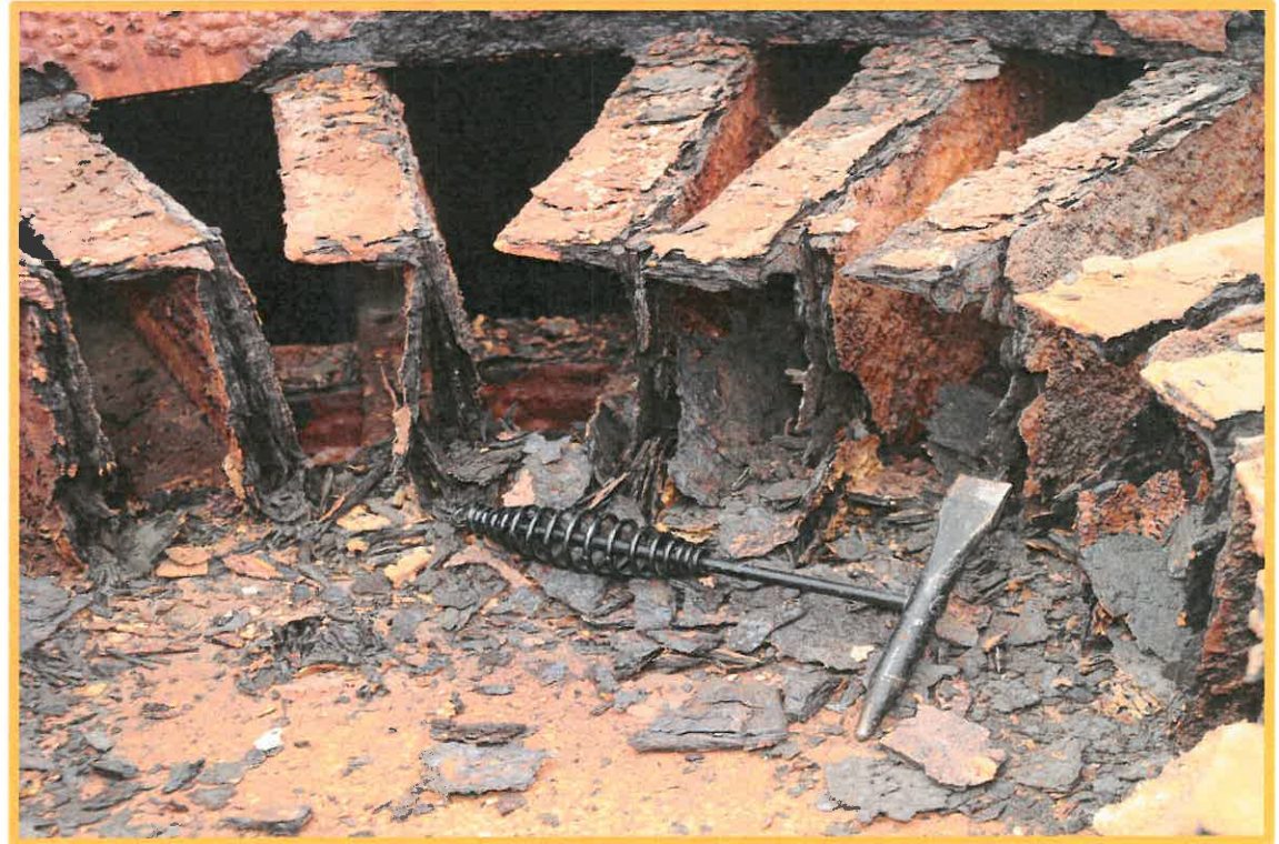
West Reservoir Center Rafters
