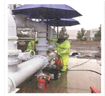
CDA Winter Maintenance Shutdown
