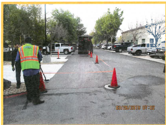
HQ Paving Safety Improvements
