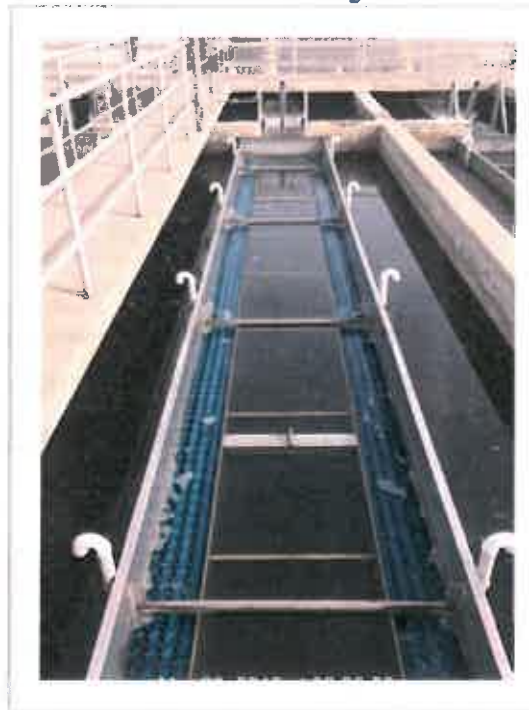
RP-4 Trident Filter Rehab Project
