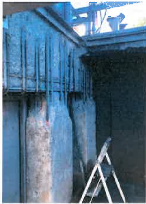
RP-1 Headworks & Primary Upgrades
