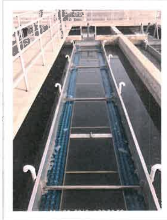
RP-4 Trident Filter Rehab Project
