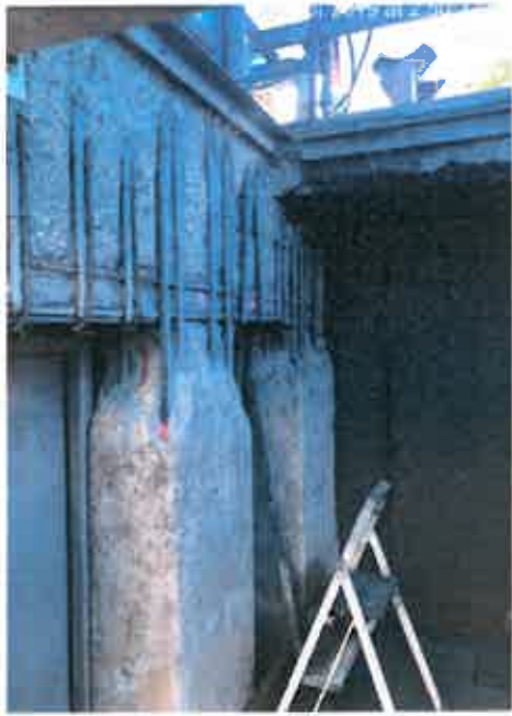
RP-1 Headworks & Primary Upgrades
