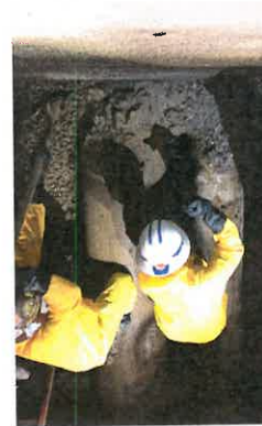
Engineering: Pipeline Repair
