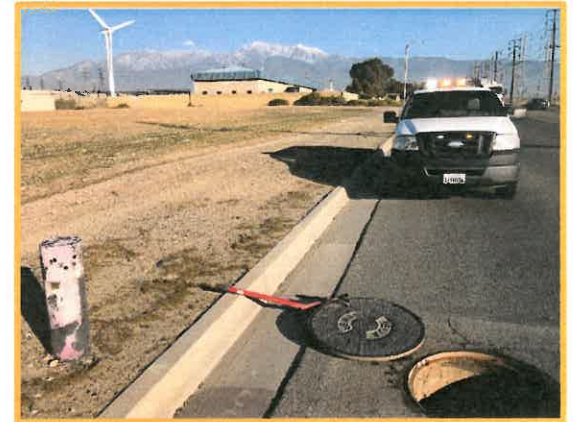
Air Relief Valve in Etiwanda Ave.
