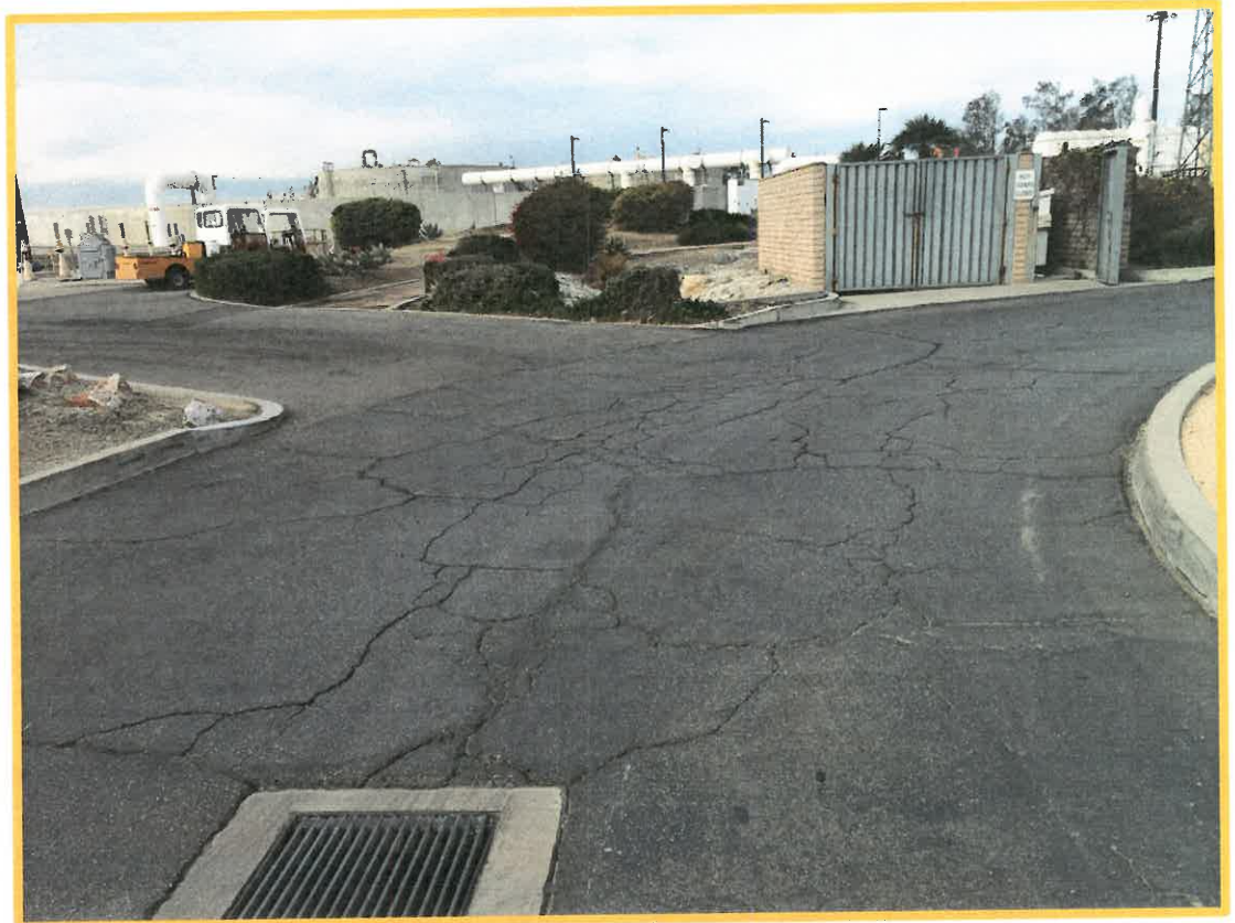
Entry to Parking Area at RP-1. Slurry Seal obscures failed A.C.
