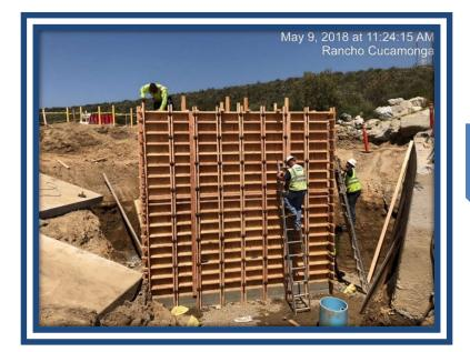
San Sevaine Project – Developing forms for the inlet structure for pump station.
