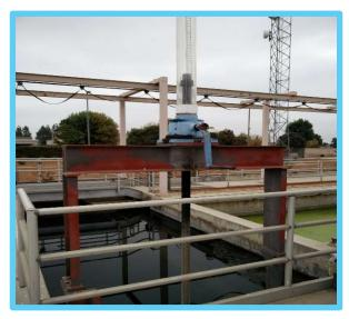
Corroded Isolation Gates at the Filters
