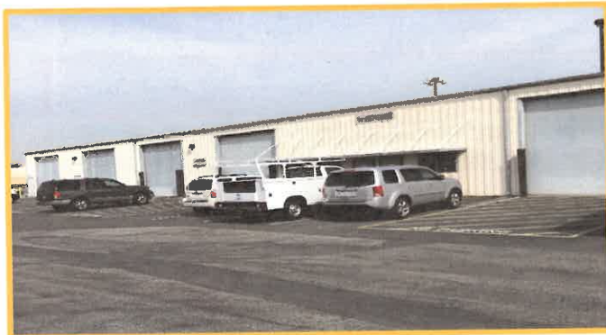
Eastside of Cucamonga Creek Channel Warehouse Building letter "R"
