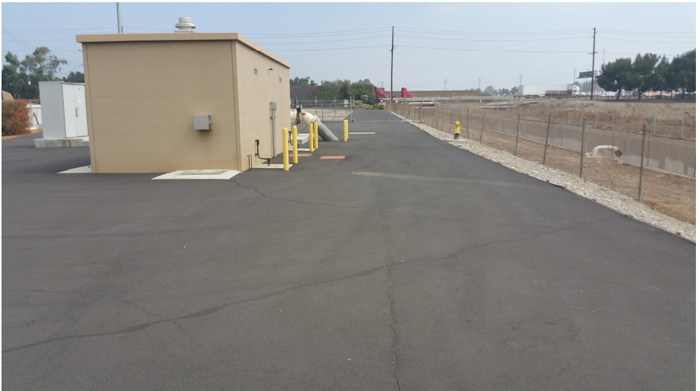
Overview of central portion of IEUA Well Refurbishment Project area (view to north)
