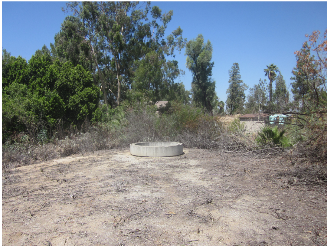
Overview of concrete pipe in central portion of WMWD Pump Station project (view to NW)
