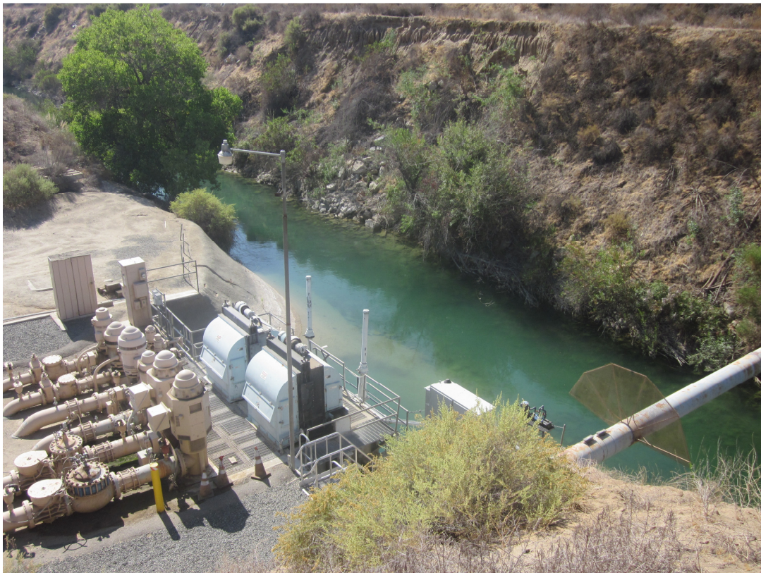
Overview of pumps and CRA crossing within ID-4 CRA Project area (view to SE)
