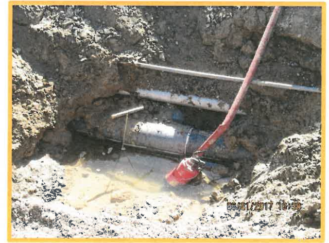
RW Pipe Rupture Repair Due to Surge
