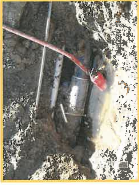
RW Pipe Rupture Repair Due to Surge
