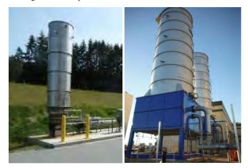
Figure 7.6-7: Enclosed Waste Gas Burners
