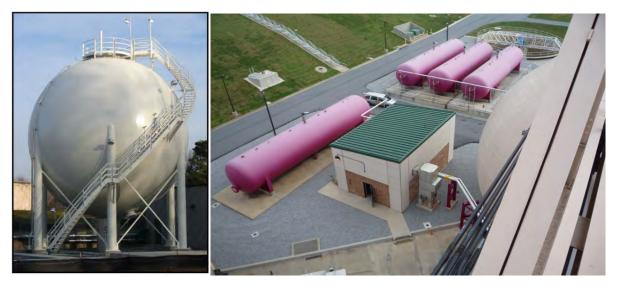
Figure 7.6-5: High-Pressure Gas Storage
