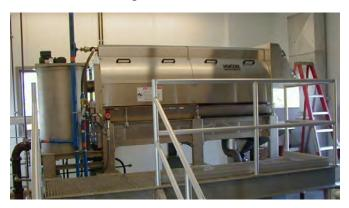
Figure 2-3: Rotary Drum Thickener
