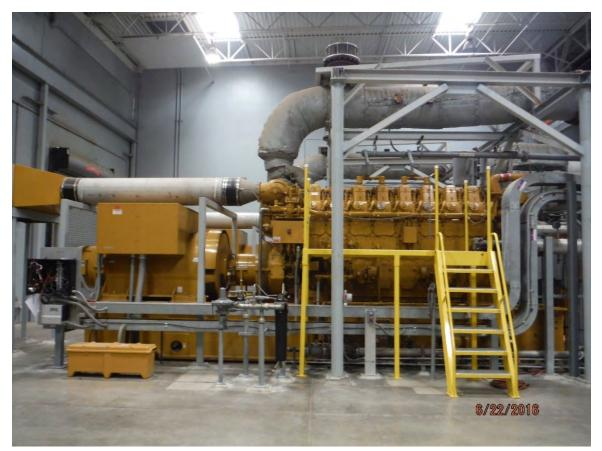
Figure 9-2: One of Two Existing Caterpillar Internal Combustion Engines
