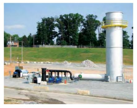
Figure 7.6-8: Ultra-Low Emission Enclosed Gas Flare
