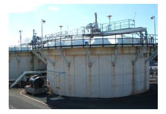
Figure 7.3-3: Gravity Thickener
