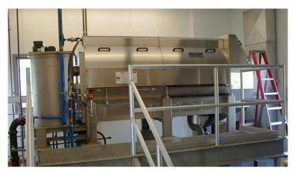
Figure 7.3-7: Rotary Drum Thickener
