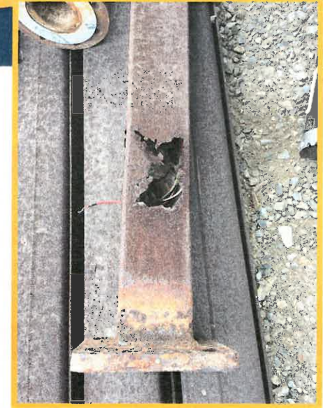
Existing Corroded Light Pole
