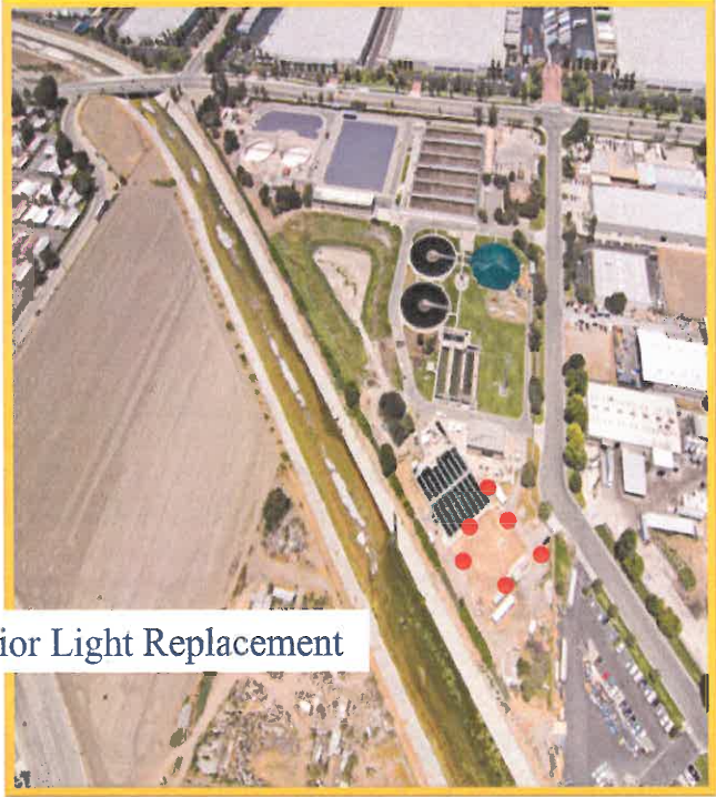
CCWRF Aerial Photograph
