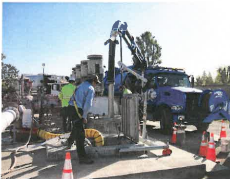
RW Pump Station Inspection
