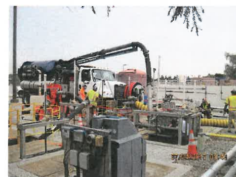
Headworks Condition Assessment
