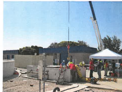
Primary Clarifier Inspection
