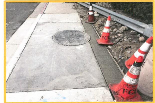
New GMI Manhole Installation
