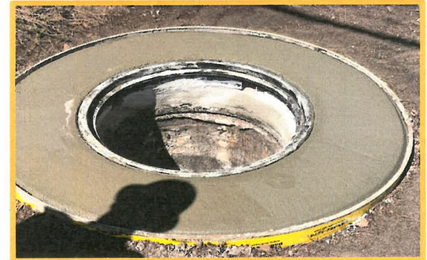
New Concrete Manhole Collar
