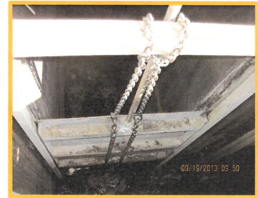
Gate Upstream of Headworks: Failed to Open
