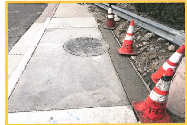
New GMI Manhole Installation
