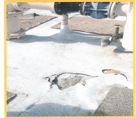
Cracking of Foam Roofing Insulation
