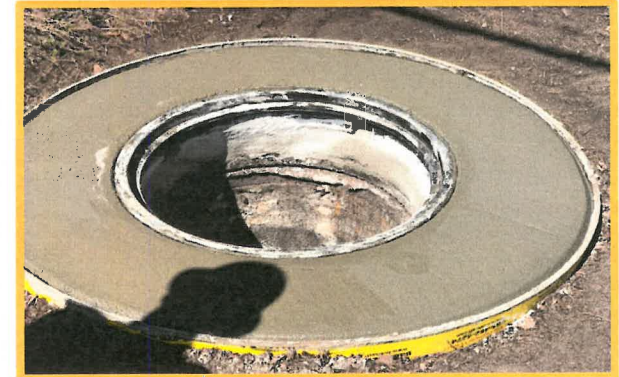
New Concrete Manhole Collar
