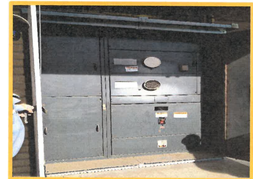
Outdated 480V Switchboard Board will be Replaced
