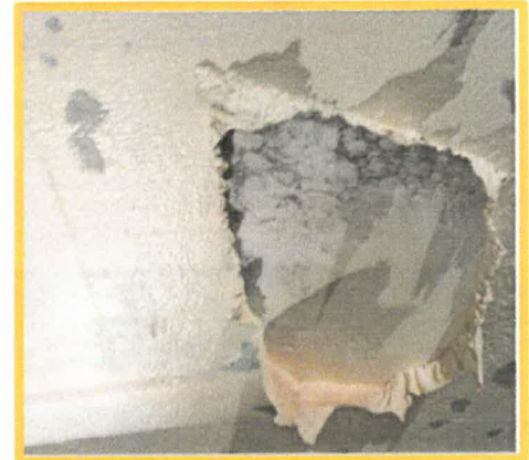
Failed Internal Roof Coating
