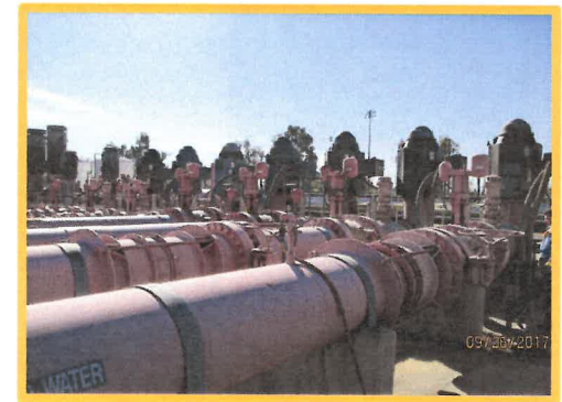
RP-1 Recycled Water Pumps
