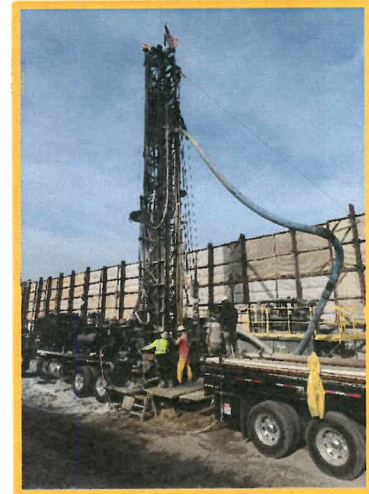
Main Rig to Drill to 350-feet
