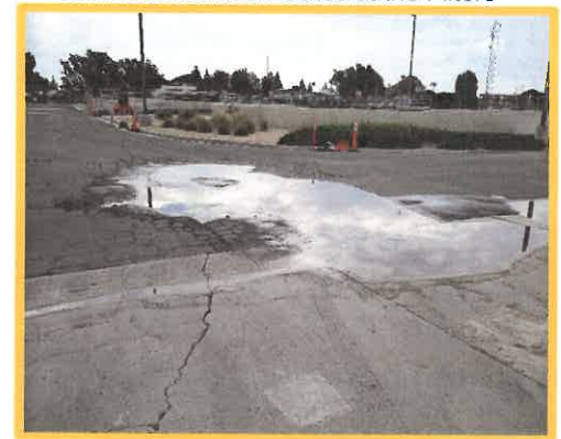
Surface Cracks and Drainage Issues
