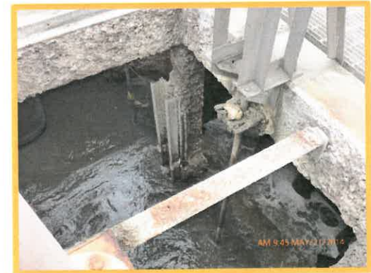
Exposed Rebar in Grating at Support Beam
