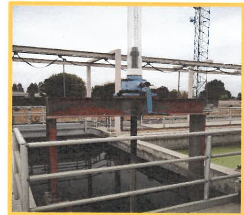
Corroded Isolation Gates at the Filters
