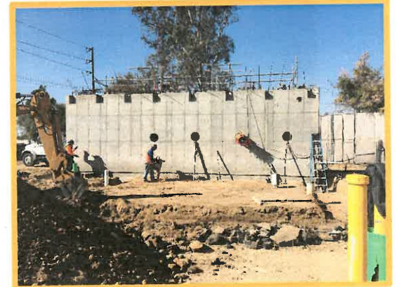
Wet Well Construction
