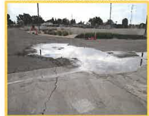
Surface Cracks and Drainage Issues
