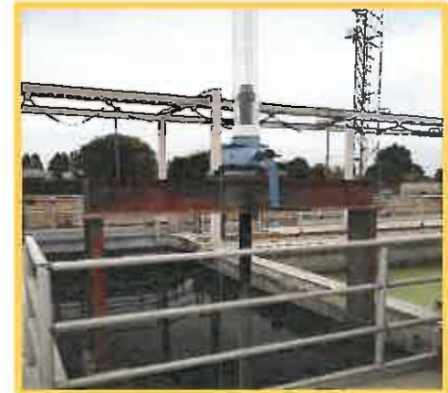
Corroded Isolation Gates at the Filters
