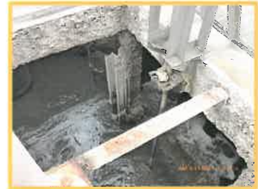
Exposed Rebar in Grating at Support Beam
