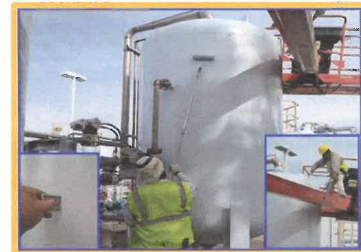
Finish Coat to Process Tanks
