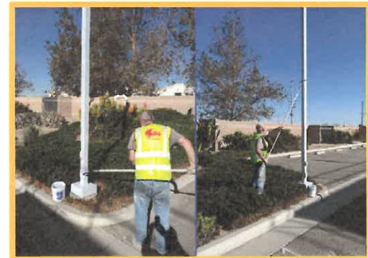
Finish Coat to Light Poles
