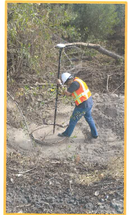
GPS Manhole Locating
