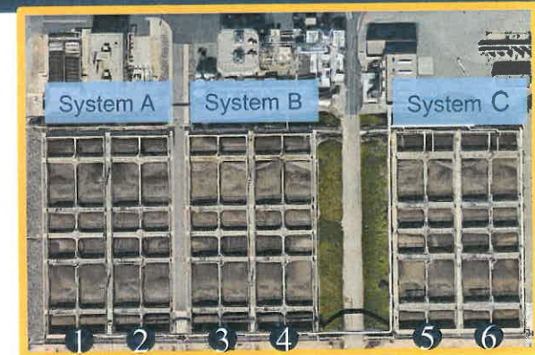
RP-1 Aeration Basins
