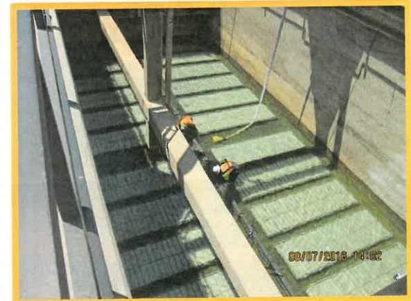
Repairing air header piping
