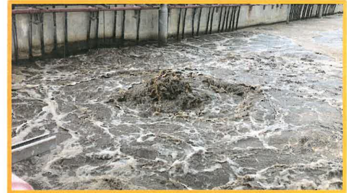
Aeration Basin Surface Boil
